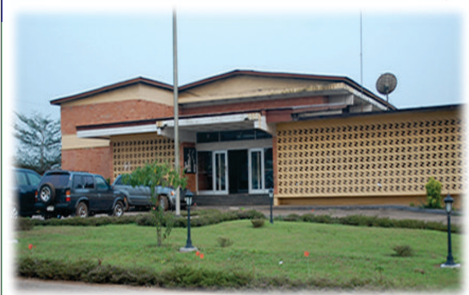
Front view of the Administrative Building
